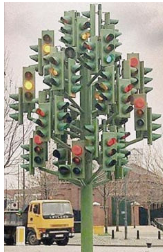
Red light spells danger: is too much precaution the way forward
